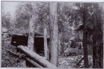
La Bale Tunnel showing Clarence Wright (second from right) as a boy.
